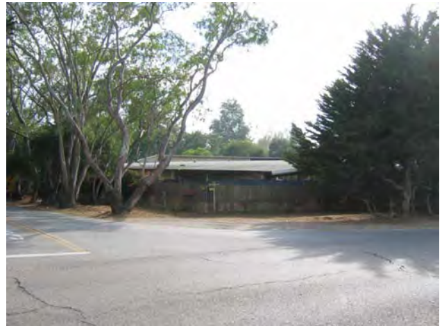
Site H from East Valley Road opposite Sheffield Drive; note floodwall surrounding property.
