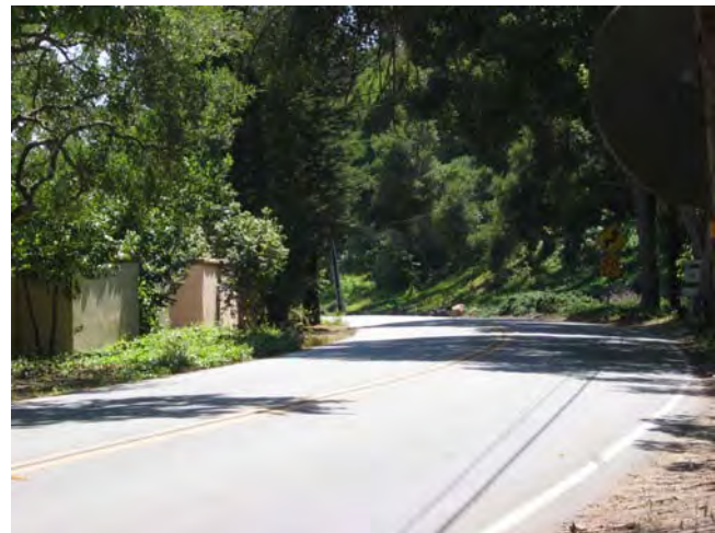
Facing south on Sheffield Drive, this curve in the road restricts line of sight and poses safety concerns.
