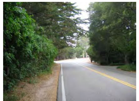
Line of sight to the west on East Valley Road from Location 1 may be an issue due to the limited line of sight and high vehicle speeds.
