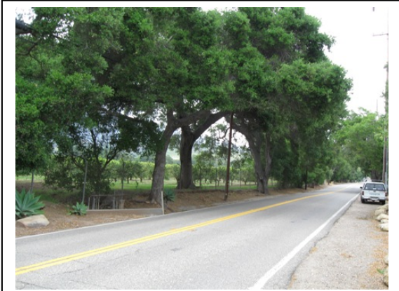
The project site is located along a straight and level stretch of East Valley Road, which affords excellent visibility in both directions.
