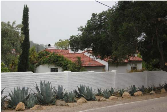
The two-story residence located south of the project site has minimal setbacks off East Valley Road.
