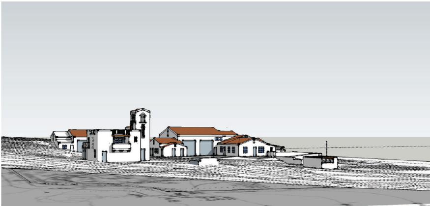
View of Main Station from Northeast
