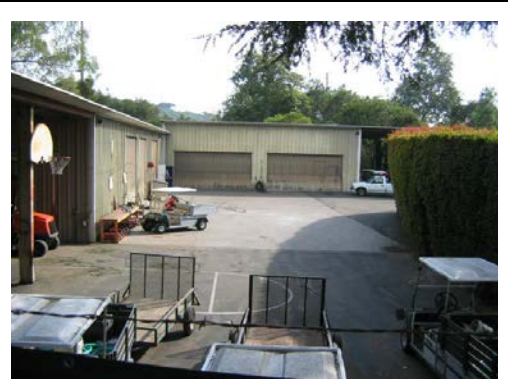
The potential site is currently used for Birnam Wood Golf Club maintenance facilities.
